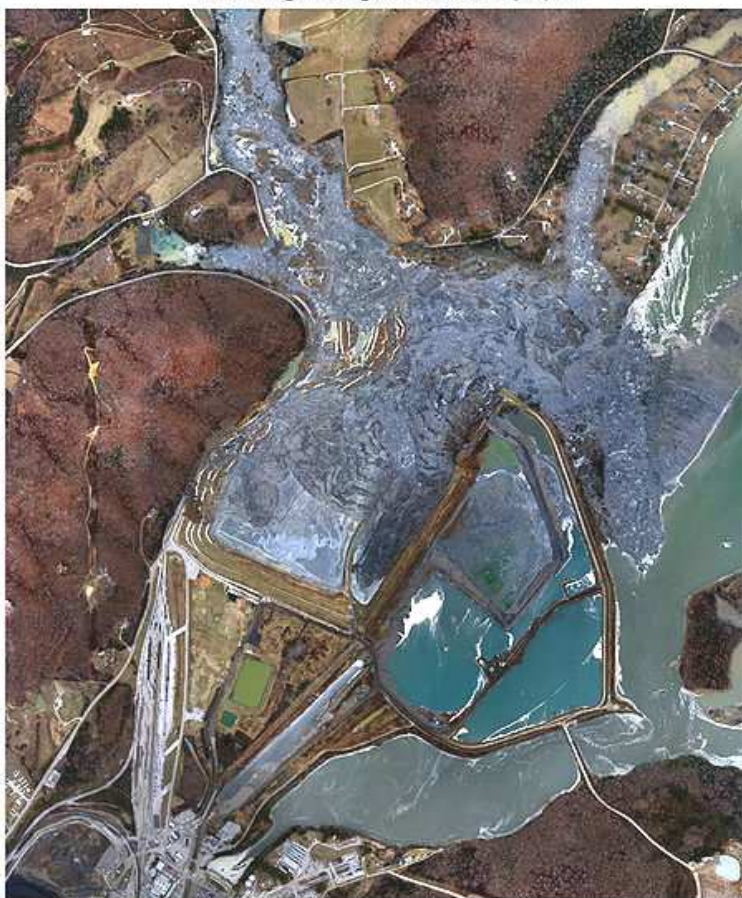
Aerial Image Of Kingston Ash Slide 12/23/08
